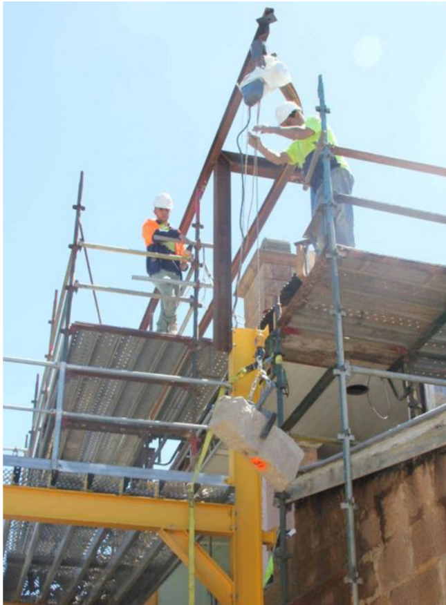
Workers deconstructing the western wall, stone by stone.
