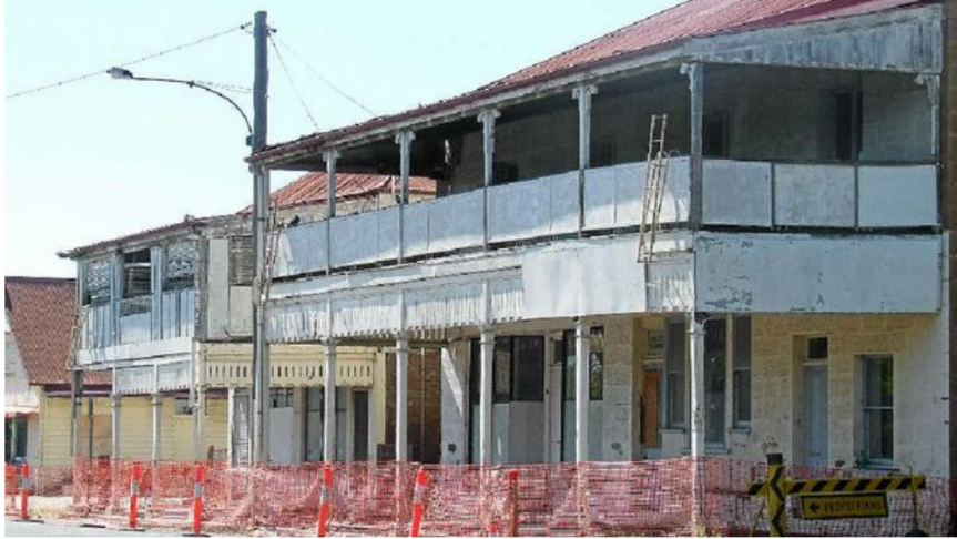
RIGHT, the building before the restoration process began.
